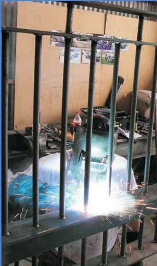
The structural steel team has provided the balustrades for the Inland Revenue's parking building in Christchurch.
