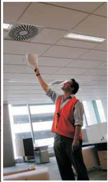
PBS manager Martin Pfaff indicates one of the FCUs, which control temperature throughout the Inland Revenue building.
