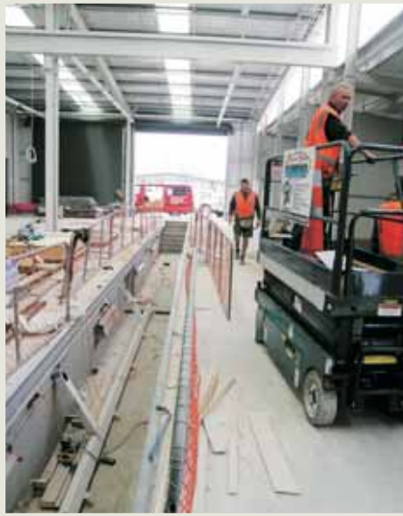
Work is nearing completion on the new truck workshop at Fonterra's Clandeboye plant.
