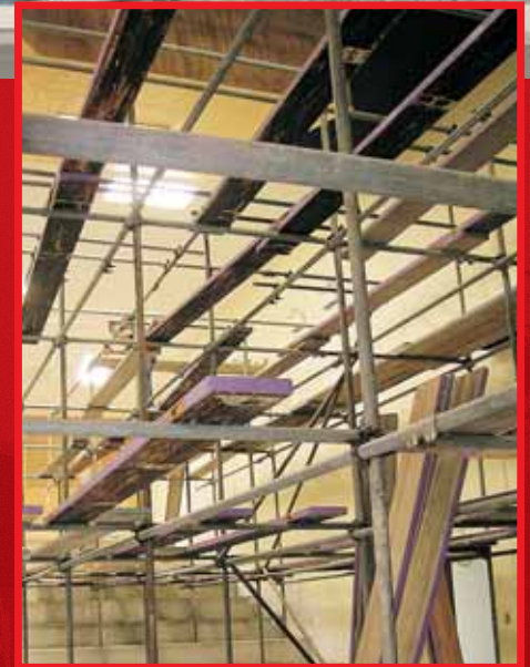
Scaffolding in place at the Craighead Girls' School auditorium.
